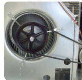
PowerMax DriveN Pulley on a Centrifugal Fan.
